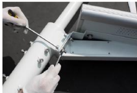
9. Fix the light on the socket by screws and insert the wind turbine cables into bracket
