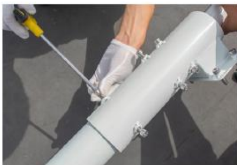
8. Insert the light pole into the connecting socket and fix it with screws
