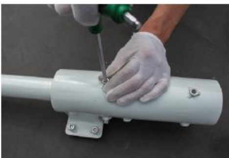
7. Fasten the three longest screws on the connecting socket
