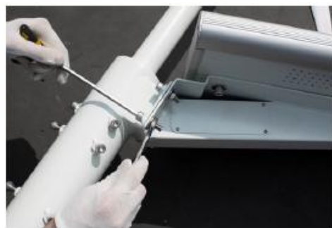
9. Fix the light on the socket by screws and insert the wind turbine cables into bracket
