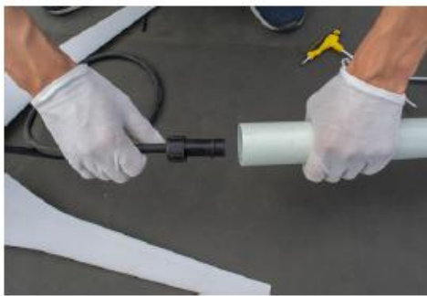
4. Insert the wind turbine cables into the connecting socket
