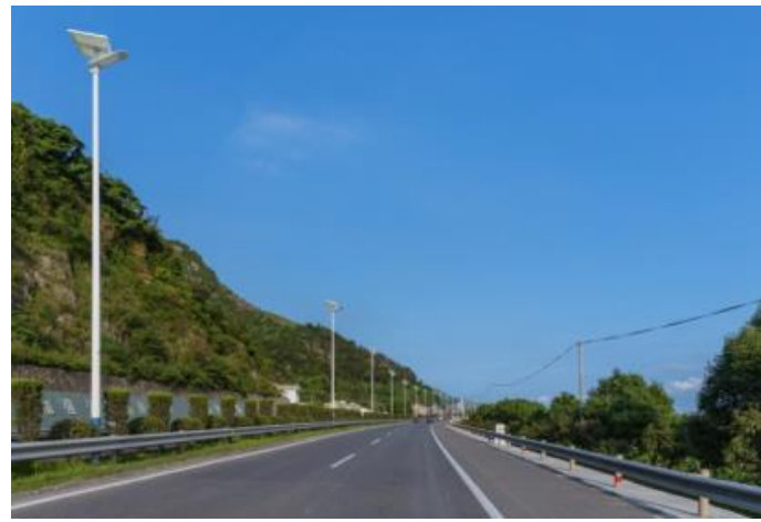
Traffic Road Lighting
