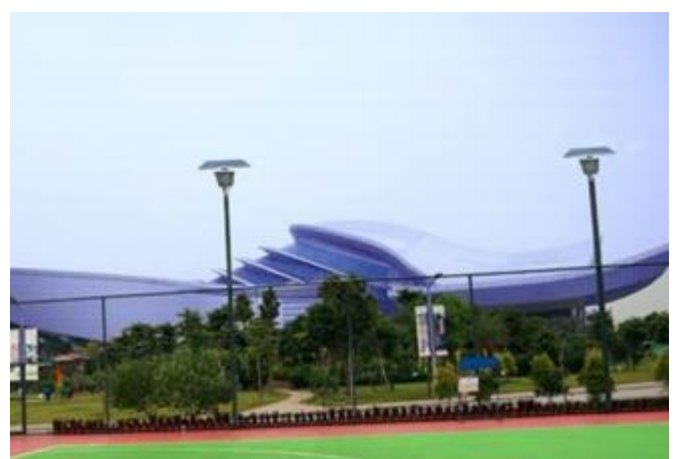
Outdoor Stadium Lighting
