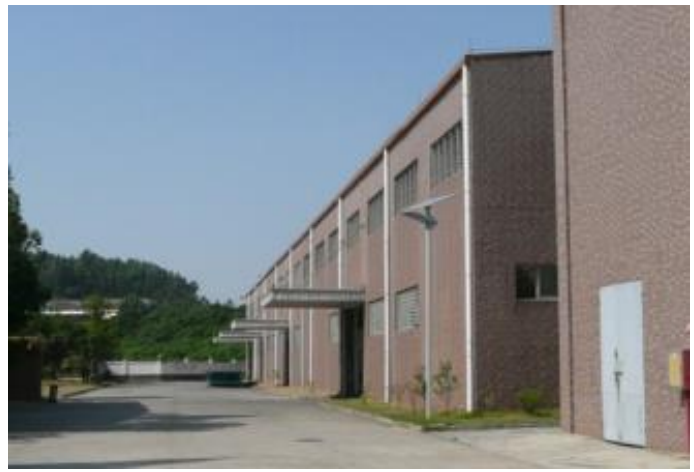
Industrial Estate Lighting
