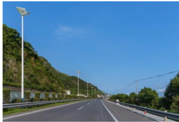
Traffic Road Lighting
