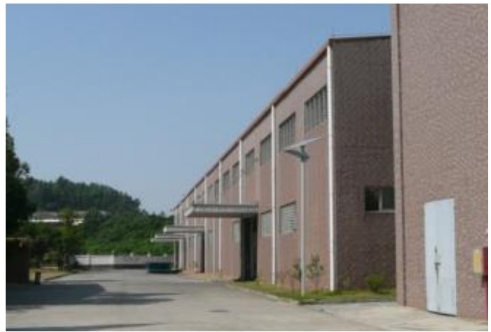
Industrial Estate Lighting
