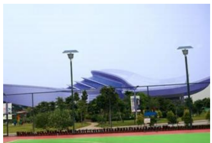
Outdoor Stadium Lighting
