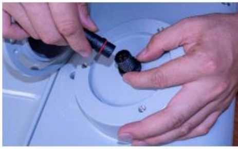
1. Connect the quadripuntal connectors of Horizontal Brackets & Light body together
