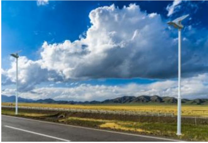
Traffic Road Lighting
