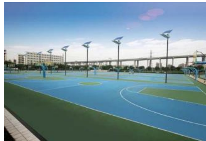
Outdoor Stadium Lighting
