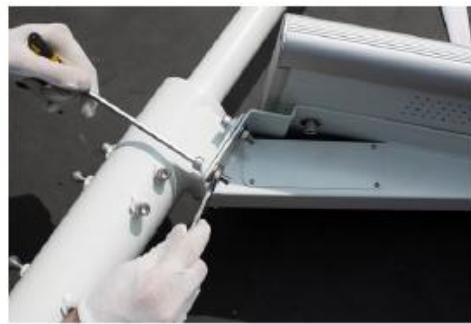
9. Fix the light on the socket by screws and insert the wind turbine cables into bracket
