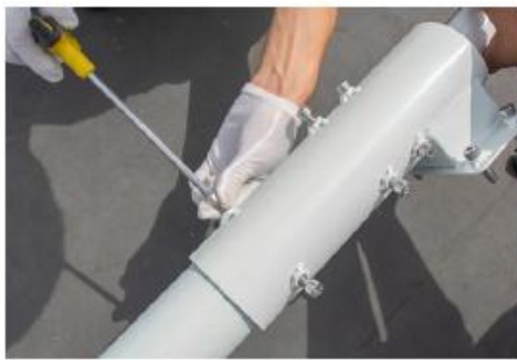
8. Insert the light pole into the connecting socket and fix it with screws
