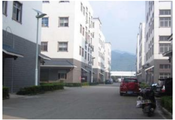
Industrial Estate Lighting
