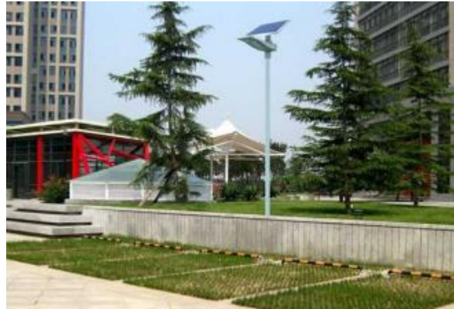
Open Parking Lot Lighting
