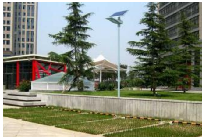
Open Parking Lot Lighting
