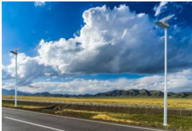
Traffic Road Lighting
