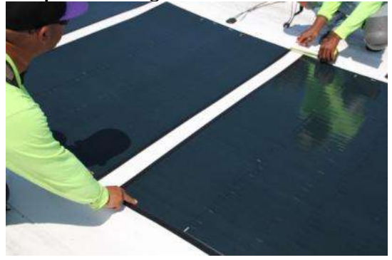
Step 4: Using roller to enhance fully bonding
