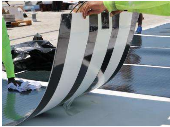
Step 3: Peeling off back adhesive tape
