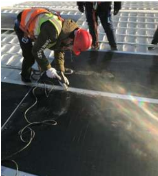
Step 4: Connect different Flex PV sheets
