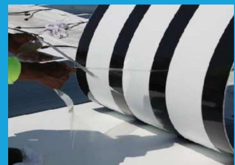
Peel & Stick Modules to Membrane
