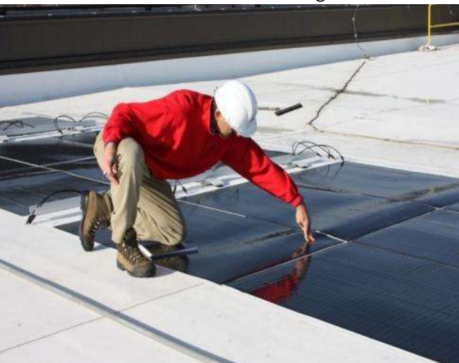
Metal Roof direct bonding
