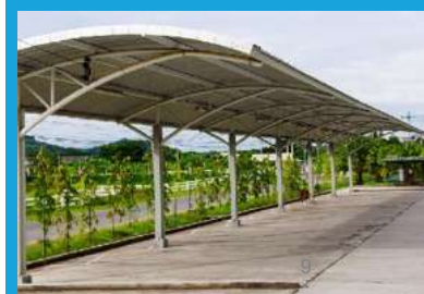
Solar Parking Canopies
